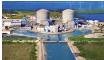
Nuclear power plant on Hutchinson Island, FL
