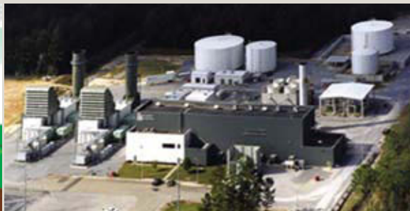
Alabama 110 MW CAES Power Plant, Alabama Electric Cooperative's McIntosh
